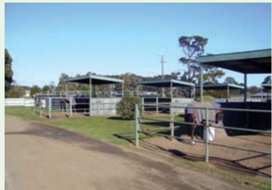
Stable yards are well laid out, tidy and maintained regularly to avoid risk of injuries due to slips, trips and falls.
